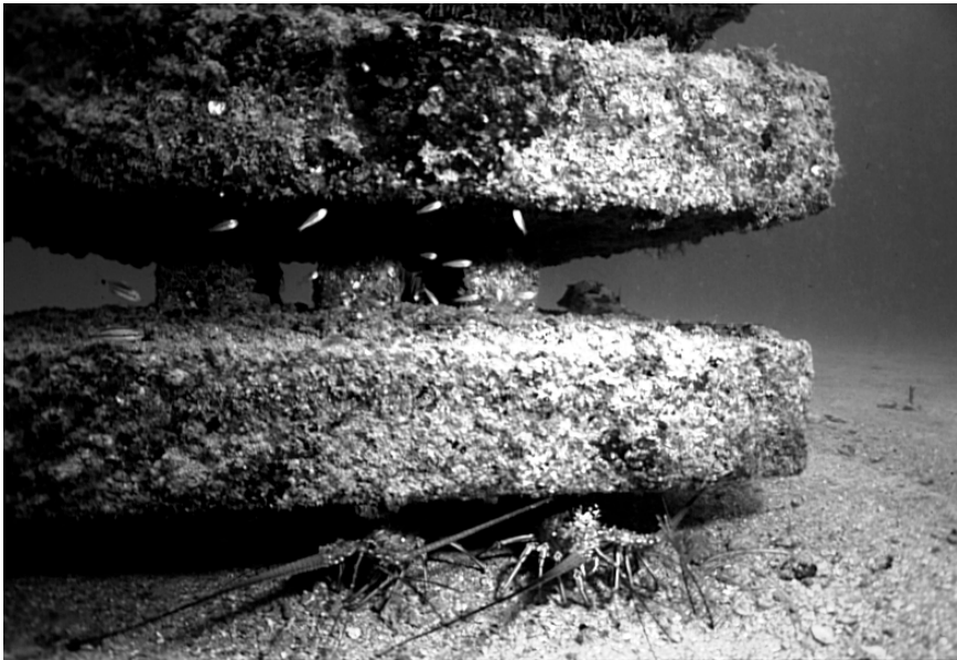
Figure 6: Example of a designed concrete artificial reef used for fish recruitment and predation studies [6].
