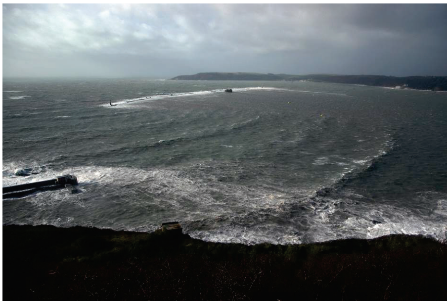
Figure 7: The Breakwater sheltering the waters of Plymouth Sound in a storm. Huge waves still make their way in through the eastern entrance showing what storm conditions would have been like in Plymouth Sound before the Breakwater was built. [The SHIPS Project]
