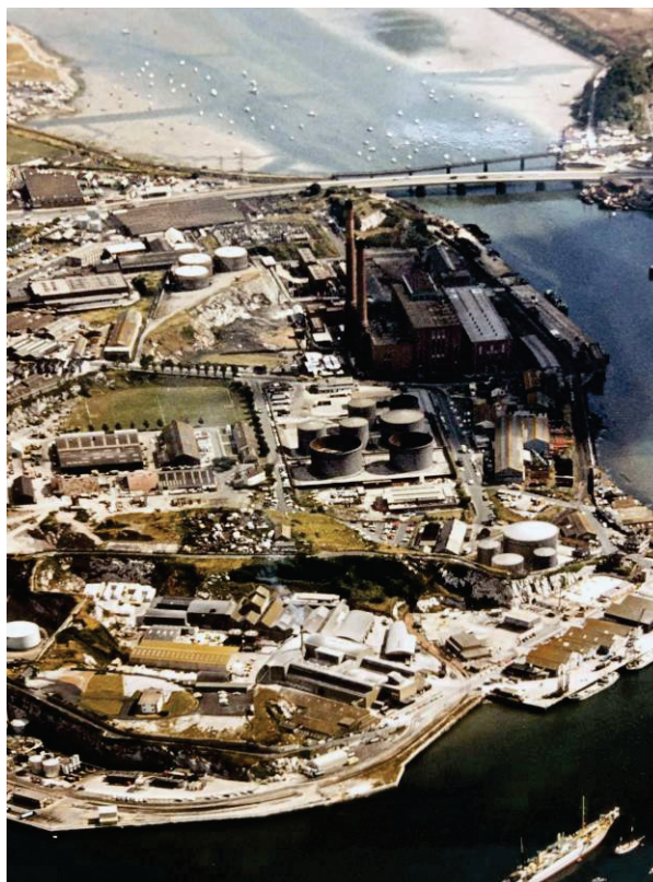
Figure 19: An aerial view of Cattedown in the 1980s from the south, showing the tightly packed factories, rail and road links, fuel storage and the power station [Cyberheritage]
