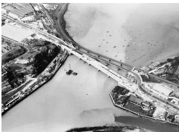
Figure 15: White china clay runoff can be seen in the river Plym in this aerial view of Laira Bridge under construction in 1961 [Cyberheritage]
