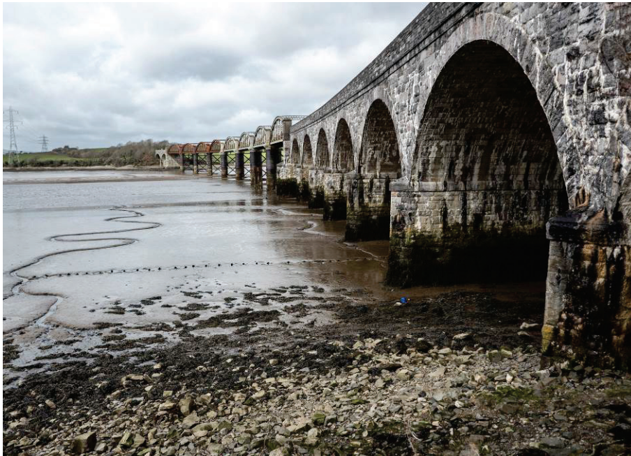
Figure 11: The railway bridge across the Tavy [The SHIPS Project]
