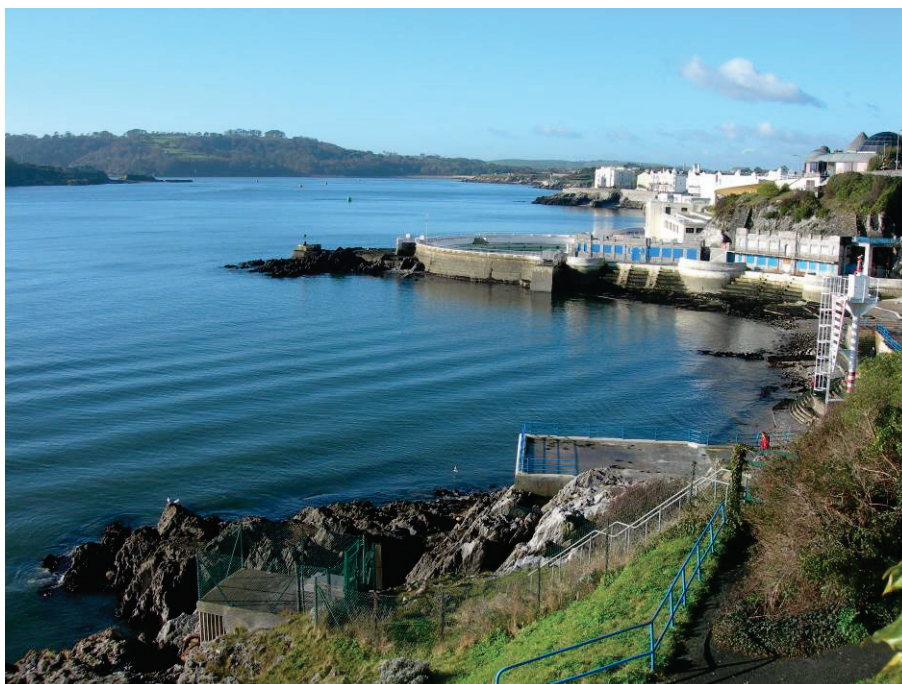
Figure 27: Plymouth Hoe foreshore with its mix of natural limestone rock outcrops and man-made structures [The SHIPS Project]
